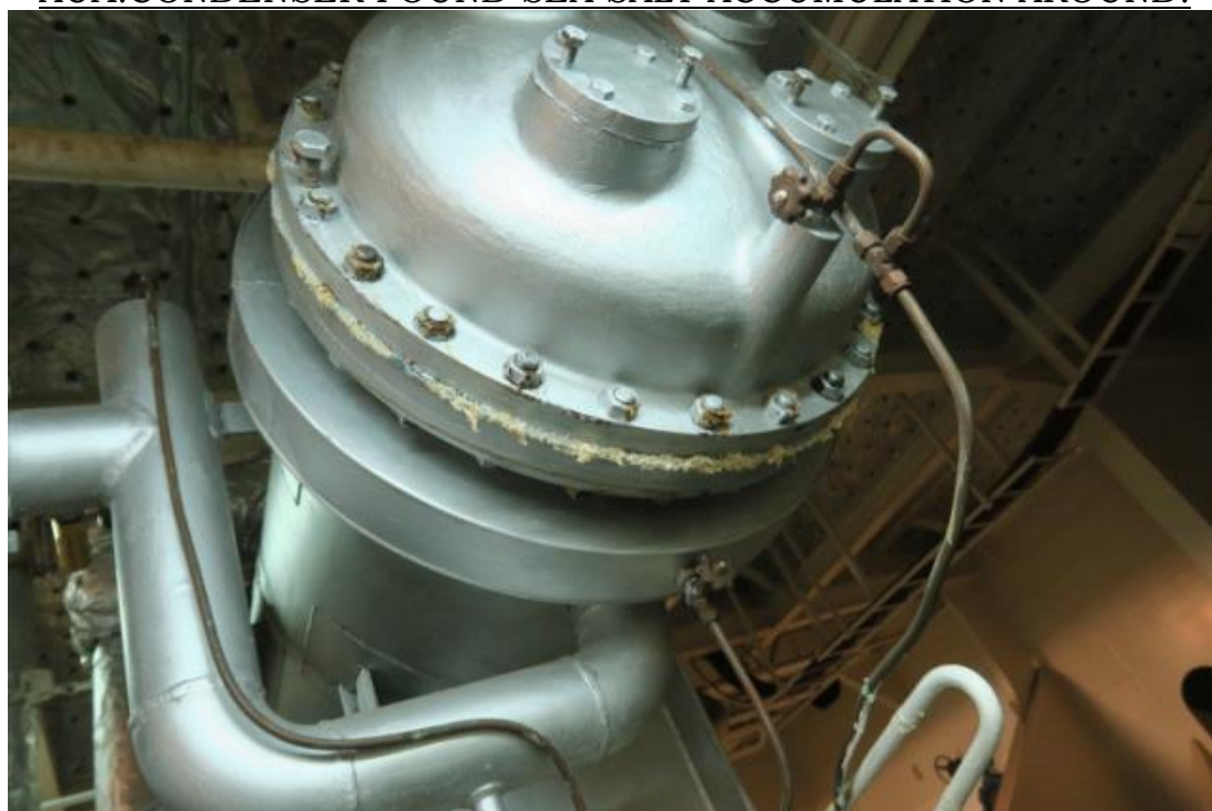
Picture of other deficiency: GASKET OF SIDE COVER FOR THE AUX.CONDENSER FOUND SEA SALT ACCUMULATION AROUND.
