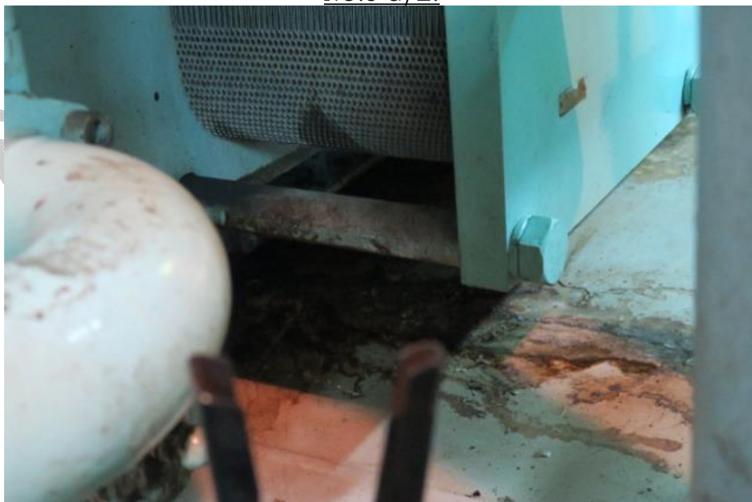
Picture of other deficiency: GASKET OF SIDE COVER FOR THE AUX.CONDENSER FOUND SEA SALT ACCUMULATION AROUND.
